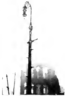
FIG. 1.—ELECTRIC LIGHT POLE.
